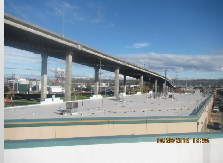
T102 Roof D
