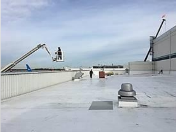
Alaska Hanger One roof
